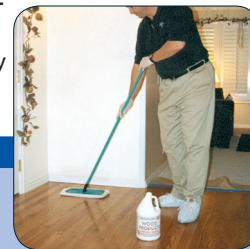
▲ Applying Wood Finish
